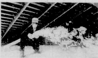
Photo illustrates Insul Safe III® Blow-In Fiber Glass Insulation. Insul Safe is thermally-efficient, noncombustible and noncorrosive for the life of a home.
